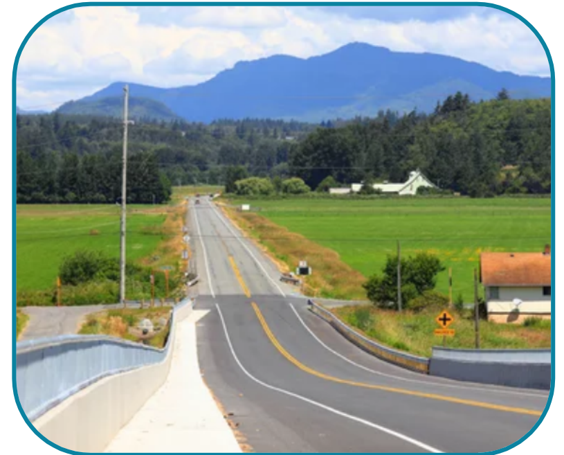
County roads not developed to urban standards
